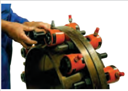
Placing cylinder and pulling nut over nut socket and bolt.
